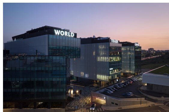
head offices of Leroy Merlin Portugal
